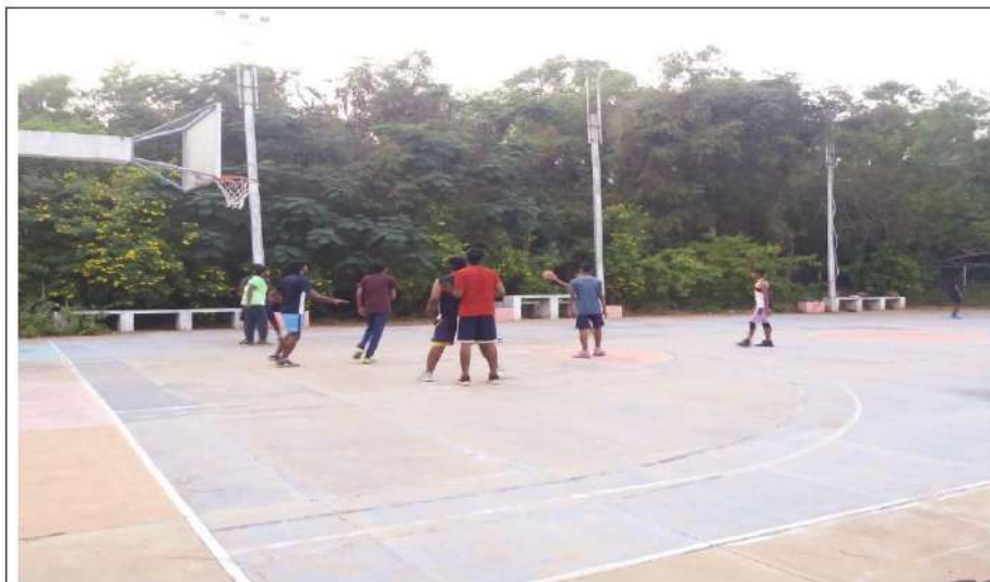
Basketball Court with concrete floor 2nos. ( Full fencing with focus light facilities )
